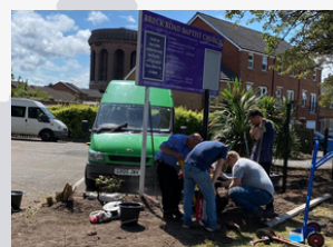
Installing the New Church Fence
